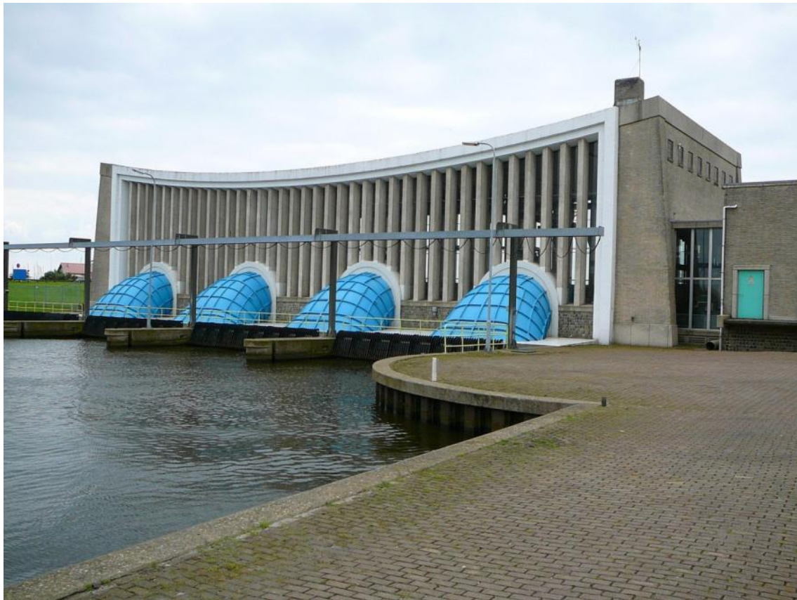
Photo 1: Hoogland pumping station (100 m 3 /s), Stavoren, The Netherlands
