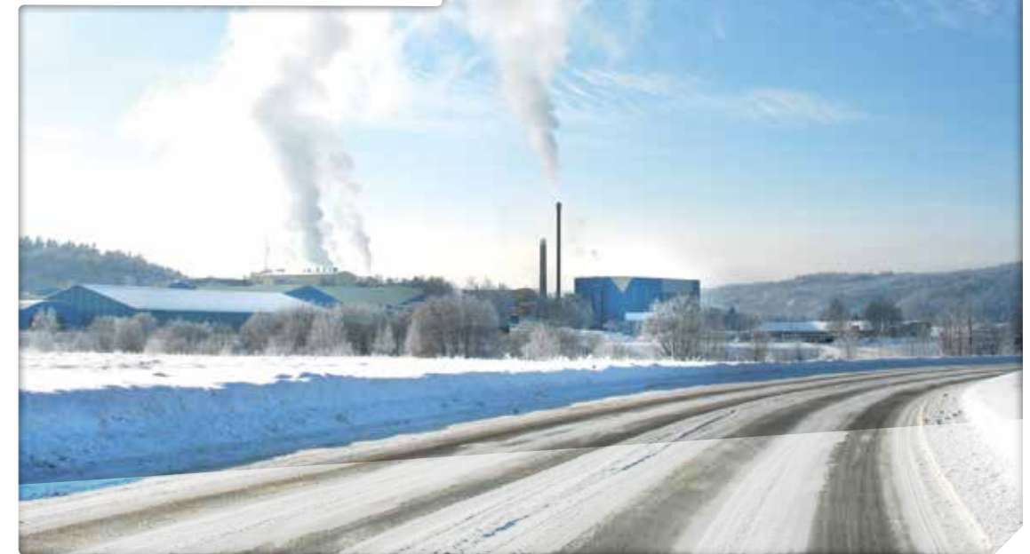
The mill at Lilla Edet no longer burns oil, but instead uses the waste from paper manufacturing and passes surplus heat on to the community.
