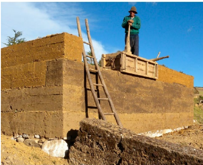
Figure 6 Traditional process for rammed earth (Recavarren et al., 2013).
