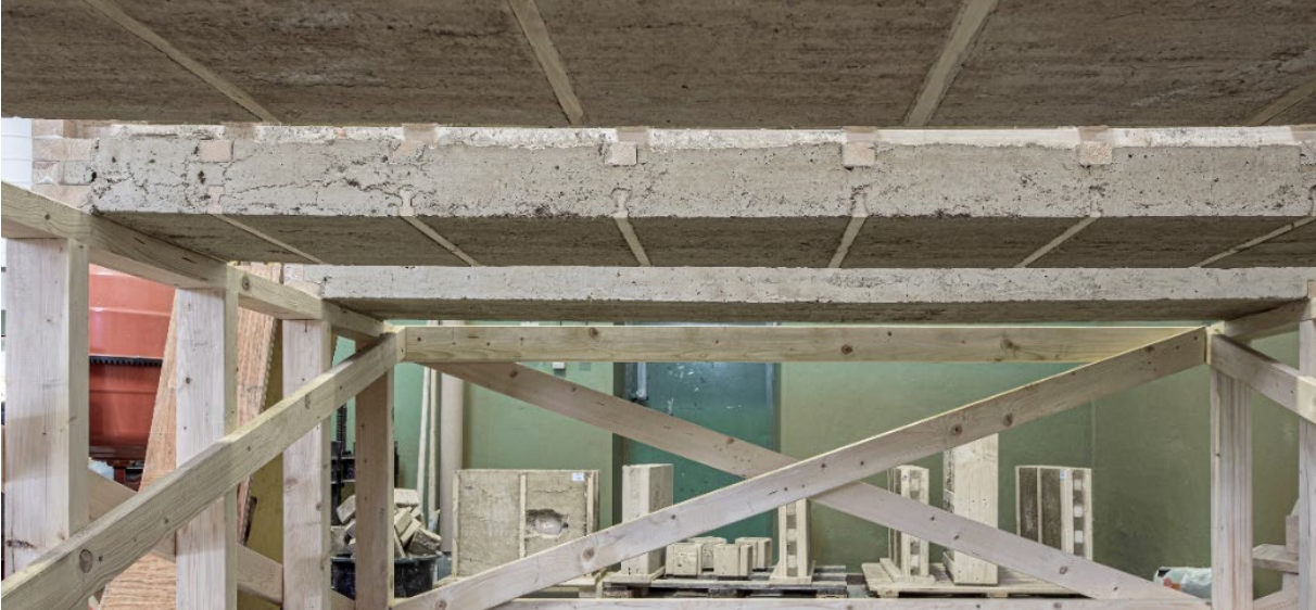
Figure 16 three prototype Hybrid floor slabs with earth infill (Trummer et al., 2022)
