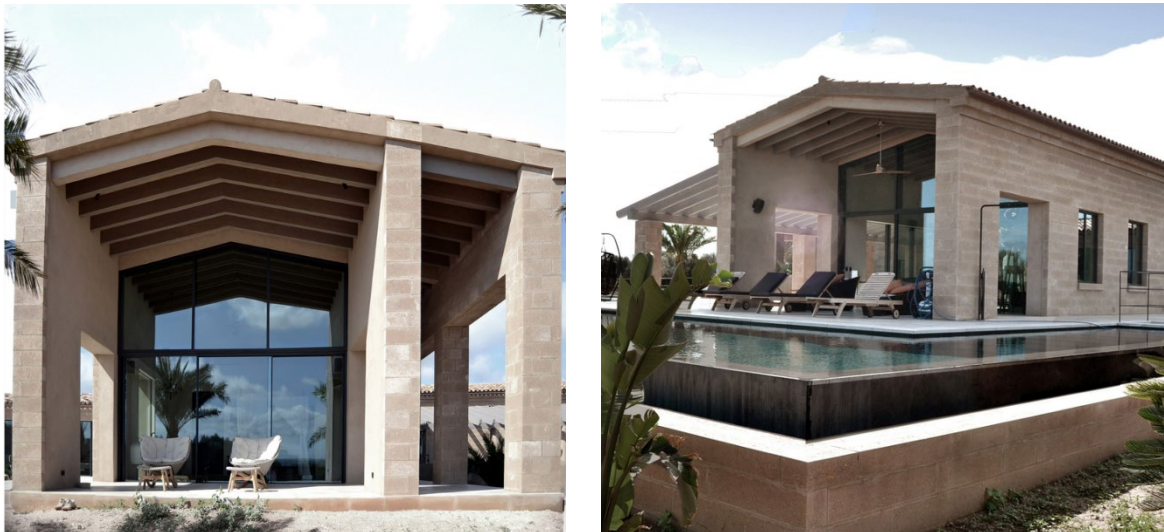
Figure 1 Finca project in Mallorca. Architects: moredesign. Structural walls for the façade with prefabricated blocks of earth Tapialblock®. All made in Mallorca with the earth of the island ( www.fetdeterra.com/en/proyecto/moredesign )
