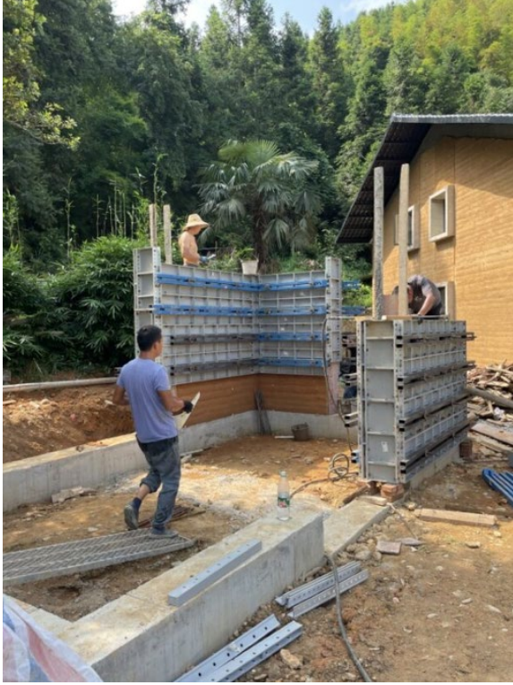
Figure 8 Rammed earth home being built Yunan Province China, 2023 (Photo: Xingda Guo)
