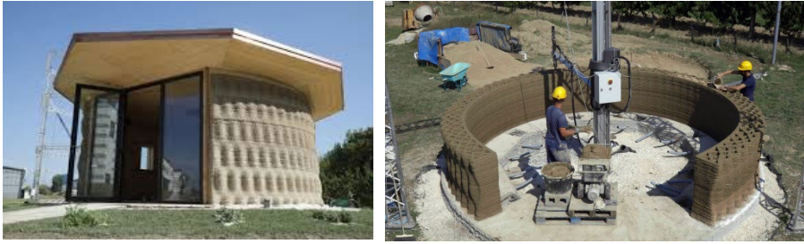
Figure 14 Printing process and the house that was built (December 2018 Gaia 3D printed earth house with Crane WASP Presentation)
