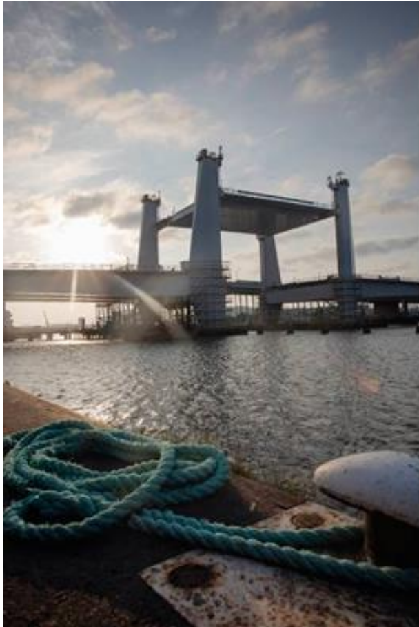
New bridge over Göta Älv river is under construction
