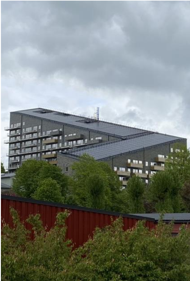
AB Framtiden building rental flats at Beväringsgatan with ecological solutions. Photo by Dan Sandén
