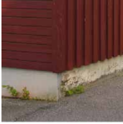
BK3-2 Concrete Slab
