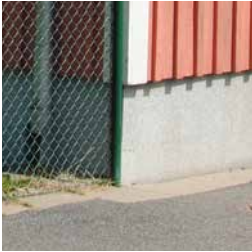
B8-1 Concrete Slab
