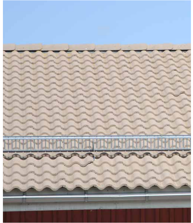
Concrete Roof Tiles
