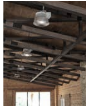
Roof construction 1.1 Structural wood
