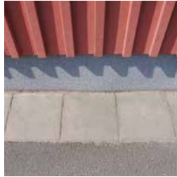
B8-3 Concrete Block
