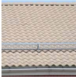
B8-2 Concrete Roof
