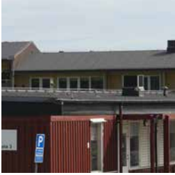
BK3-1 Asphalt Roofing
