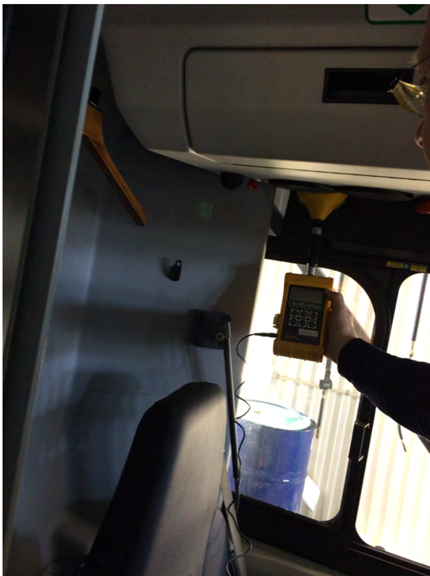
Figure 3.2. Measurement point at the cable duct, close to roof.
