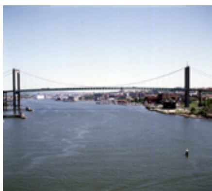
Search areas for future river crossings. Search areas also exist for future development areas, business areas, wind energy, green spaces and recreational areas.
